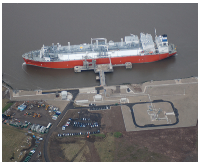
Figure 15 FSRU docked at Teeside terminal, UK
